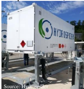
Compressor and Storage (500 & 1000 bar)
